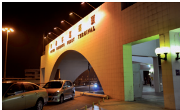
▲ Like the facility in Hong Kong, the Outer Harbour Ferry Terminal serves both ferries and helicopters.
